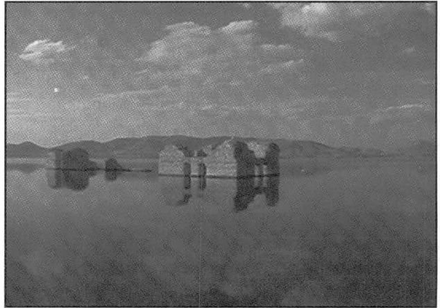
Fig. 3: The gate-houses which flanked the city gate and were built 20 m. apart on an east-west axis (Photo: by Dr. Çiğdem Özkan Ayygün)
