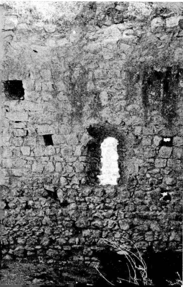
Res. 44 Kızıl han: zemin katta tonoz başlangıcı ve taşıyıcı kemer yerleri Kızıl han: vaulting system and traces of supporting arches in the ground floor
