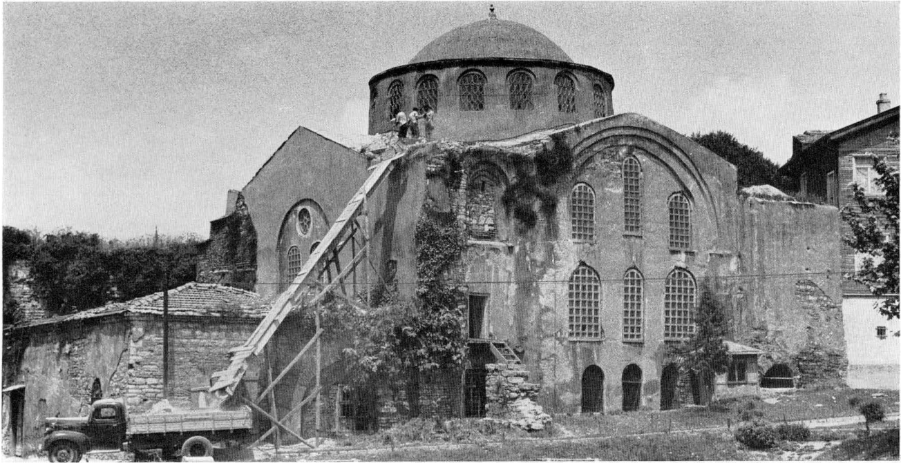
1. General View from Southwest
